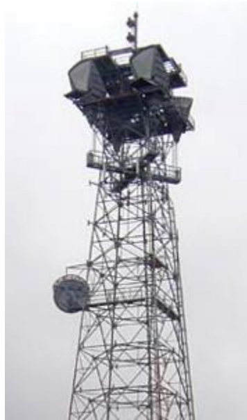
Microwave Horns on an AT&T tower. 107 were spaced across the country about 30 miles apart, receiving and re-transmitting radio signals to the next tower.
